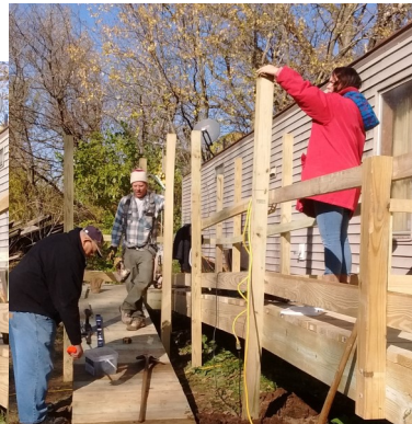
Work on the Colfax ramp
